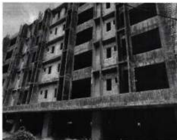
Fig: Construction at the site
